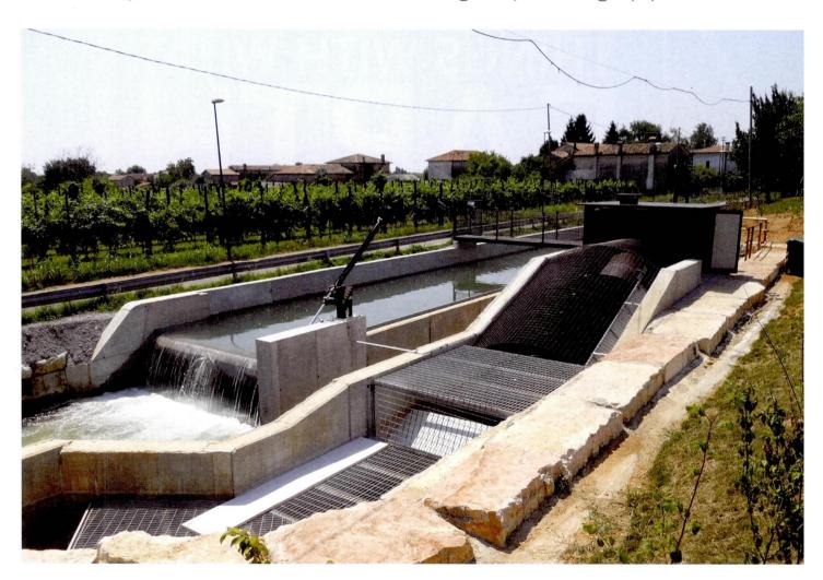
YDROSCREW IS manufactured by WAMGROUP's Italian sister company Roncuzzi and is an environmentally-friendly and cost-effective reversible volumetric machine designed for the production of electrical energy by converting hydro energy into mechanical energy. WAM South Africa general manager, Emilie clean water discharge in wastewater treatment plants, utilisation of water power in channels and for process water in paper and water milling applications.
